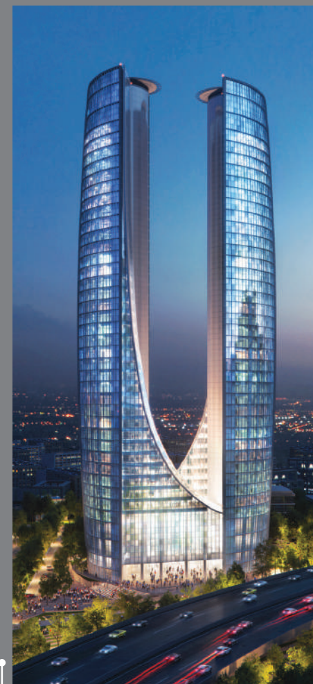
Saman Faraz Administrative towers
