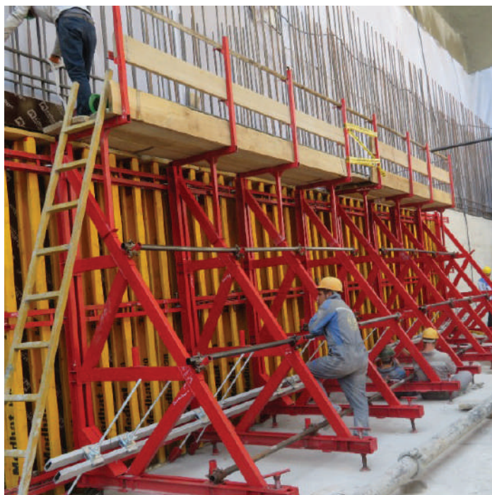
Saman Faraz Administrative Towers
