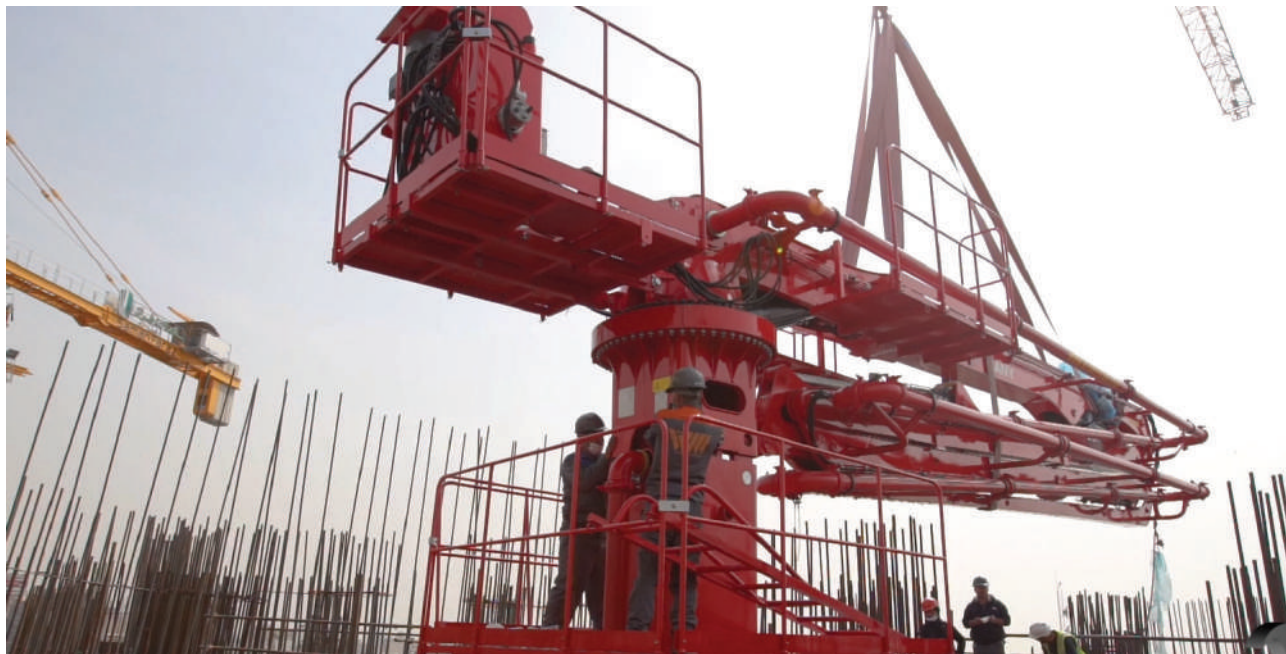
Saman Faraz Administrative Towers
