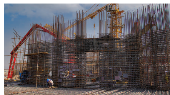
Saman Faraz Administrative Towers
