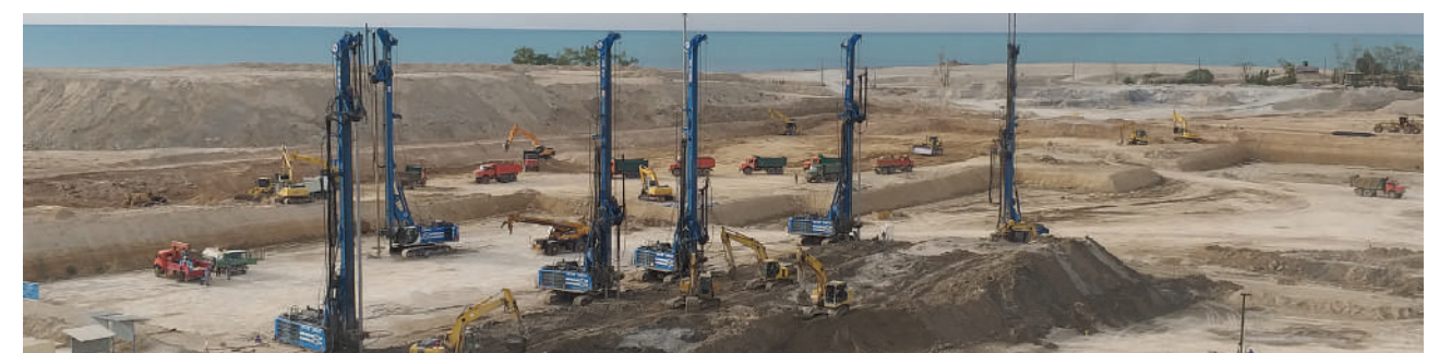
Bushehr soil stabilization project
