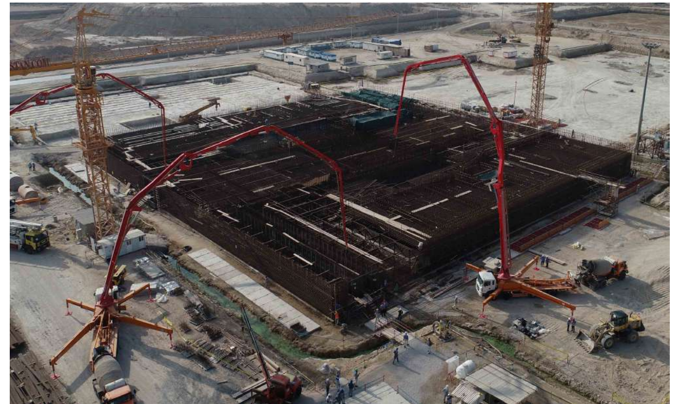
Bushehr soil stabilization project
