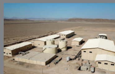
Coal-fired power station of Tabas First Coal-fired power station in Iran
